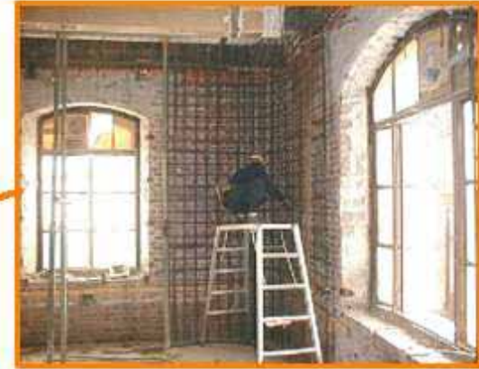
煉瓦壁RC添え打ち補強(配筋状況) Reinforcement of brick walls
